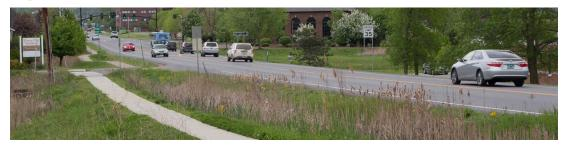
Design and construction phase services for a 242-ft sidewalk in a highly commercial area of Williston. The new 5-ft-wide concrete sidewalk is being designed to match the existing connecting sidewalk while considering the existing roadside drainage swale and bordering stormwater detention basin. The design accommodates steep side slopes on either side of the walkway.
