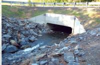
D&K developed preliminary engineering, final design, and contract documents to reconstruct this a 1.3 mile road on the existing alignment. D&K's scope of services included field survey; development of line and grade; partial relocation of the adjacent stream; streambank stabilization; permitting; coordination with VTANR and USACOE; culvert design; right-of-way acquisition. The project was cost-shared between the Towns, the State, and FEMA.
