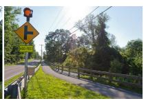
Alternatives analysis and design of a one-mile-long, 10-ft-wide bituminous bicycle and pedestrian path. D&K developed a path and landscape design that satisfied owner concerns and minimized impacts to historic properties. Due to a number of historic properties along the path alignment, this project required extensive coordination with the VTrans Historic Preservation Officer and property owners.
