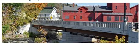
Design for replacement of a 2 span 159 ft long bridge. Superstructure was replaced using continuous horizontally curved steel beams with a composite concrete deck, and new sidewalks on both sides. Concrete bridge railings were considered a historic resource and were heavily deteriorated to the point where replacement was the only option. SHPO approved the use of the Texas Classic rail. Maintained traffic with a temporary bridge during construction.
